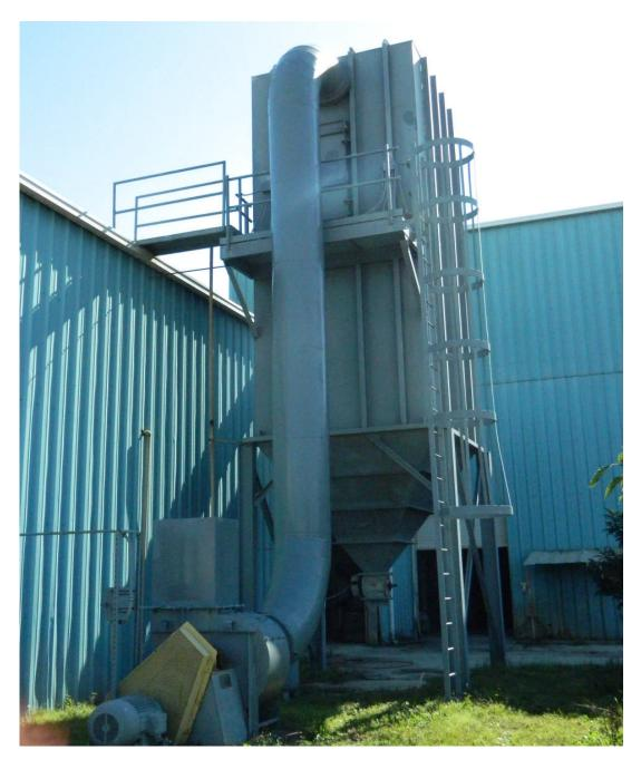
Fabric filter dust collector having 2185 square feet of filter area. Uses 168 polyester filter bags (5" diameter x 10 ft. long). 14,000 CFM using Robinson 240J 30HP fan operating at 2473 RPM (6.4:1 air to cloth ratio). Pulse cleaning, 80 gallon air accumulator included. Commissioned in 1986. Asking \$8500 (original price \$47,000).
